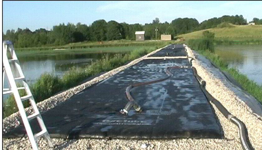
In August 2009, Six Geotube® units were used to dewater and contain sludge pumped from one of the three sewage lagoons operated by The Municipality of Arran-Elderslie.
